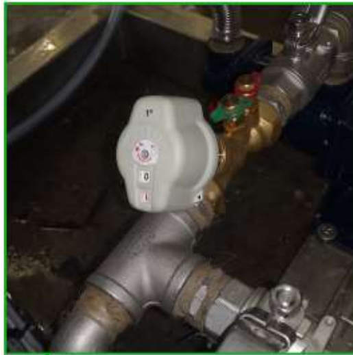
DILUTED REGULATING VALVE The valve regulates the flow of dilute into the sludge - OPEN-
